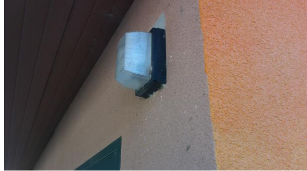
24w or 48w CFL wallpack common on portables
