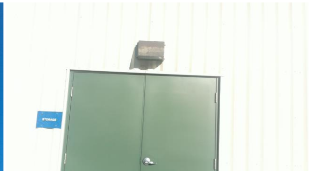
42w Quad pin CFL wall packs
