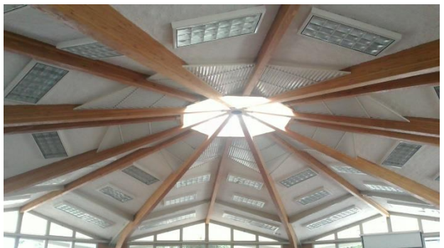
3 lamp parabolic troffer fixtures in the library
