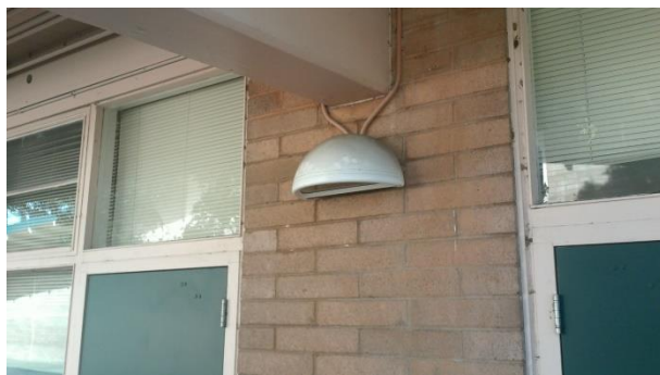
70w HPS half circle cut off wall pack
