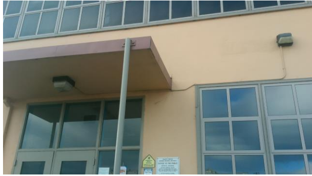
50w HPS wall pack and canopy fixtures
