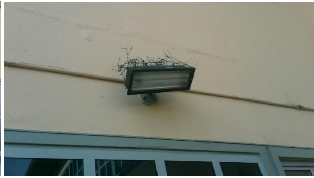
2 lamp pin based CFL flood
